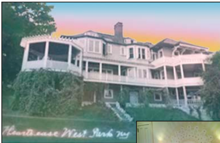
The historic Hearts Ease mansion is newly renovated and overlooks the Hudson River in West Park, NY.
